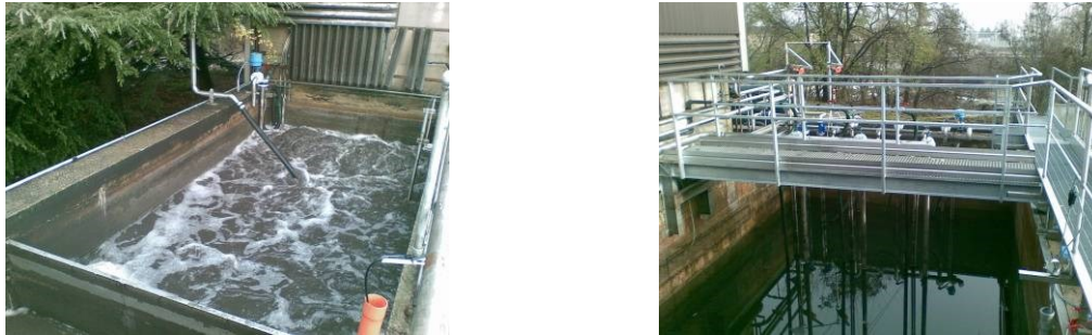
Fig. 1. (Left) iMBR plant for Low Load operation. (Right) iMBR plant for High Load operation.
