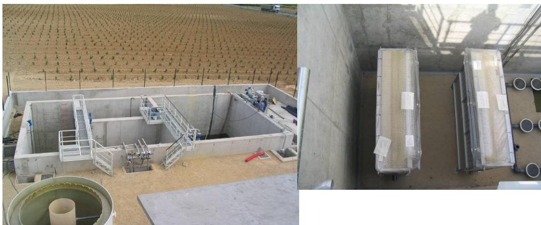
Fig 2. (Left) Modular iMBR plant under construction. (Right) Kubota Submerged Membrane Units.
