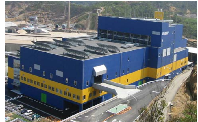
Teshima waste melting plant
