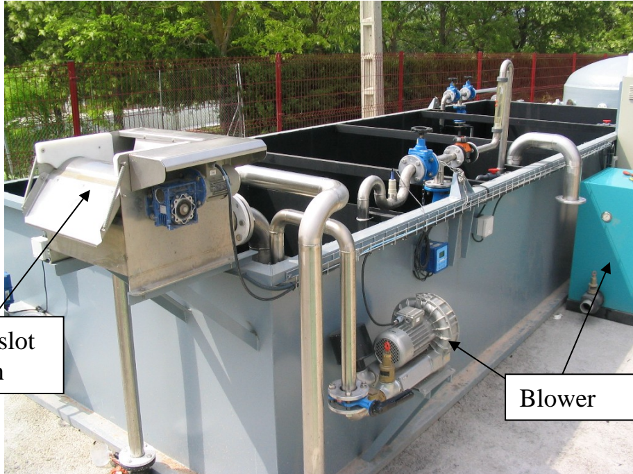
Configuration 3: NEW BUILD Buffered compact MBR plant (15m 3 /day)
