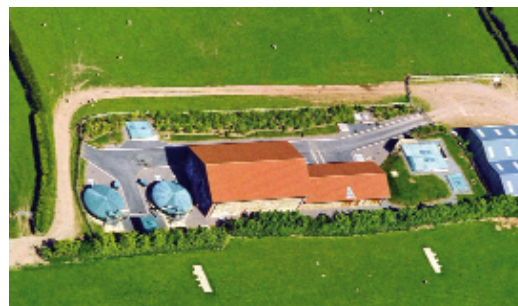
The Porlock MBR treatment plant.
