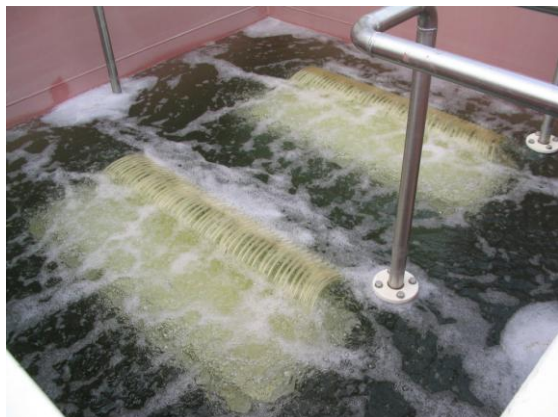
Fig 2.- Detail of the membrane reactor.
