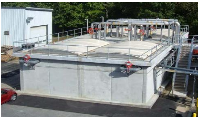
Photo of the four covered AnMBR tanks(left) and the membrane units inside the tank (right)
